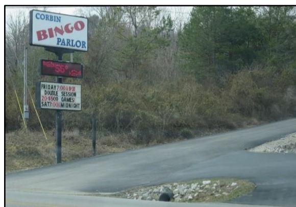
Project will rebuild entrances like this one to improve safety
