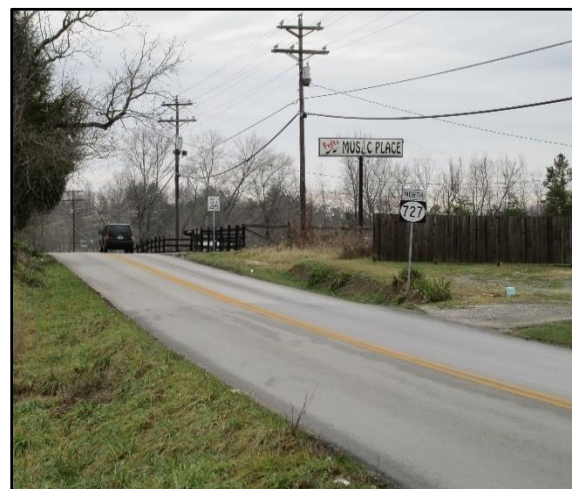
Segment 2 lacks proper sight distance
