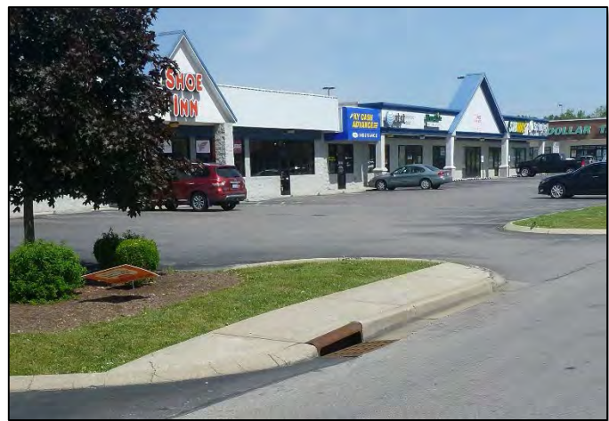
Figure 4.4 Example of disconnected sidewalk, on Dons Drive.
